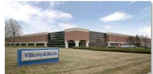
3 South Middlesex Avenue, Monroe, NJ
