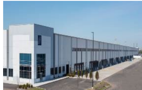
586 Gulf Avenue, Staten Island, NY
