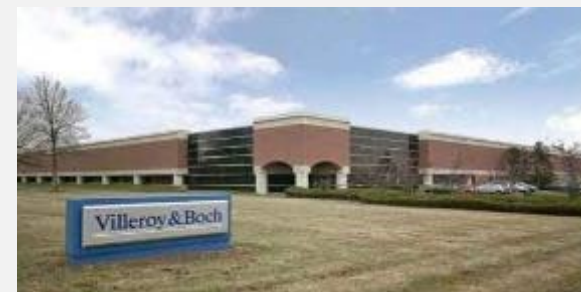
3 South Middlesex Avenue, Monroe, NJ
