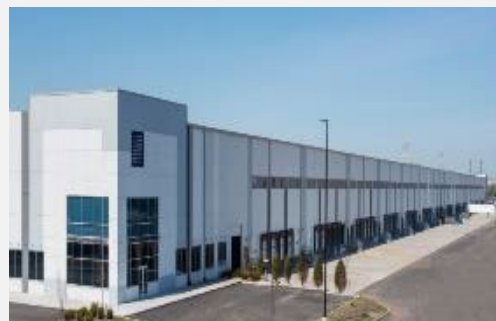
586 Gulf Avenue, Staten Island, NY
