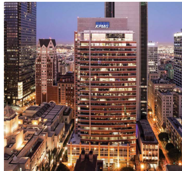
550 South Hope Street, Los Angeles, CA
