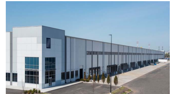
586 Gulf Avenue , Staten Island, NY
