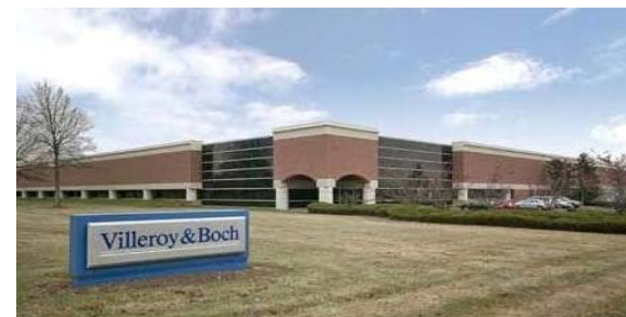
3 South Middlesex Avenue, Monroe, NJ
